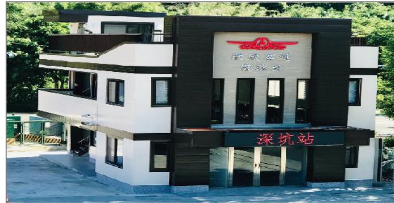
Fleet Management and Green Energy Station Monitoring Center
