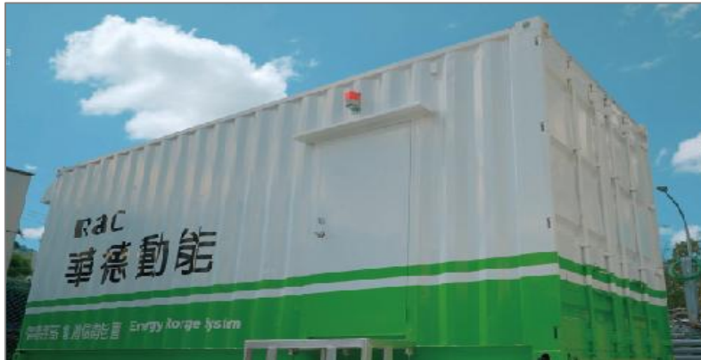
Retired lithium-ion battery energy storage system
