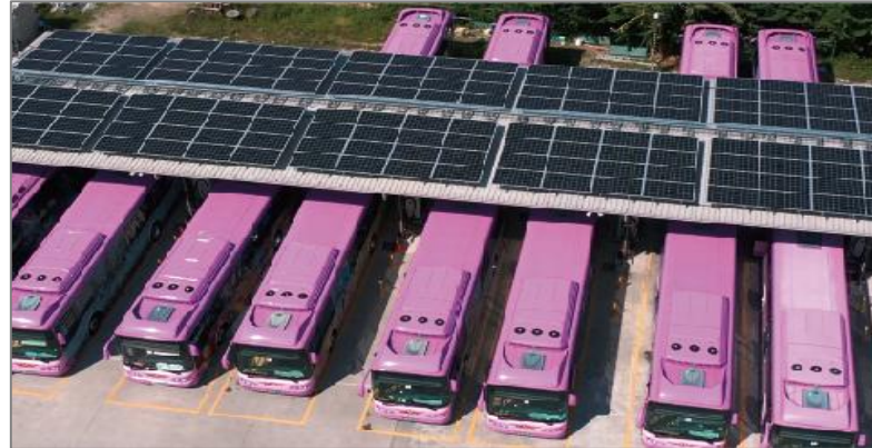
Solar power generation system
