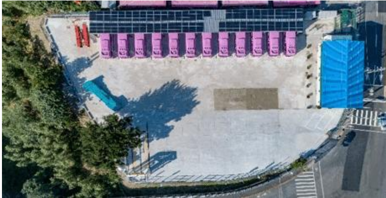
Design and Construction of EV Charging Stations Muzha / Shenkeng / Beitou
